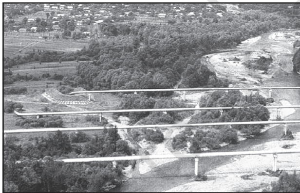
Fig. 8.17: Pipelines transporting natural gas in Ukraine
