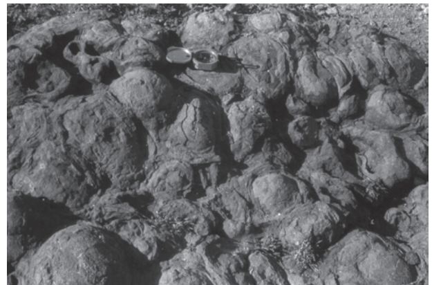
Fig.6.3 : Exfoliation (Flacking) and granular disintegration
